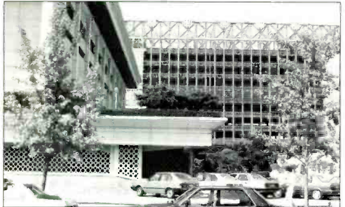
The International Broadcasting Center in Seoul, under construction adjacent to KBS headquarters.
